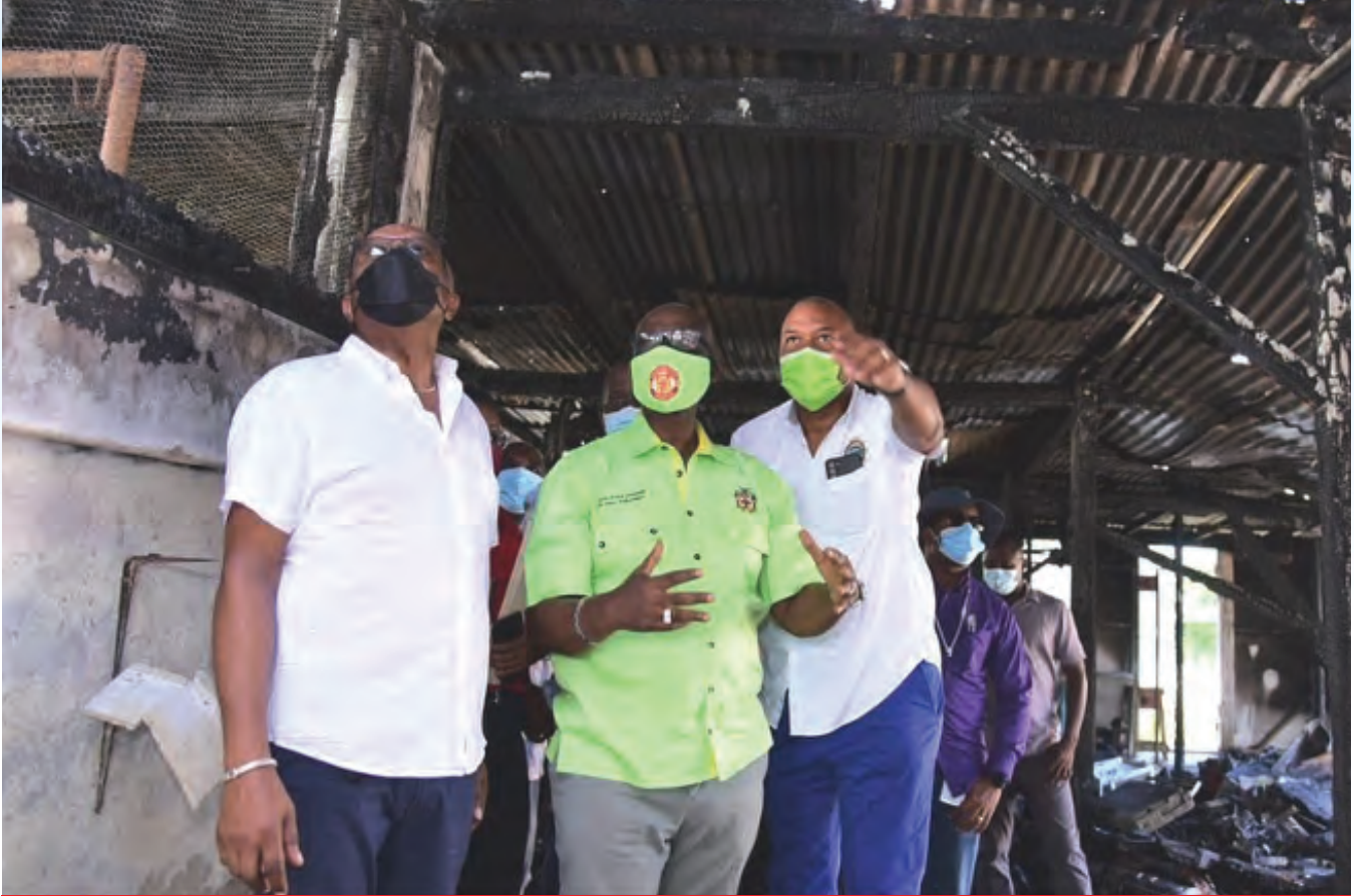
Tour of the Highgate Market which was destroyed by fire.
