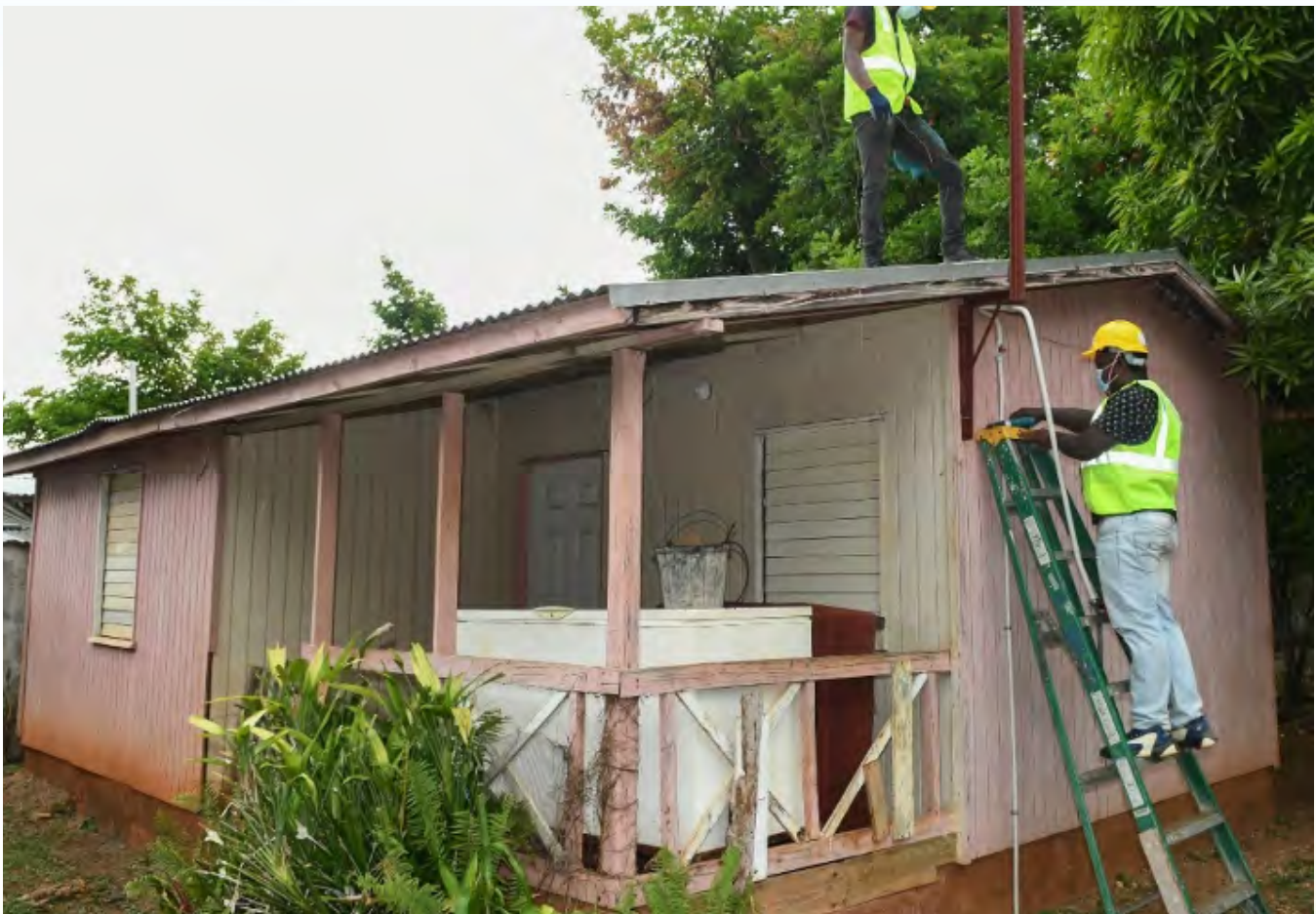
House wiring project.
