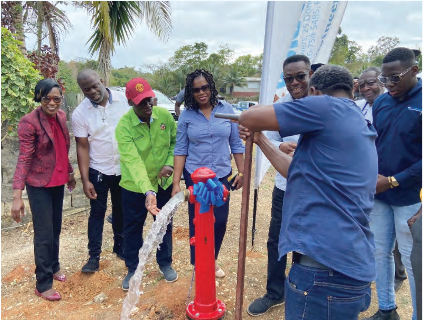
Commissioning of the Chambers Pen Water Supply System.
