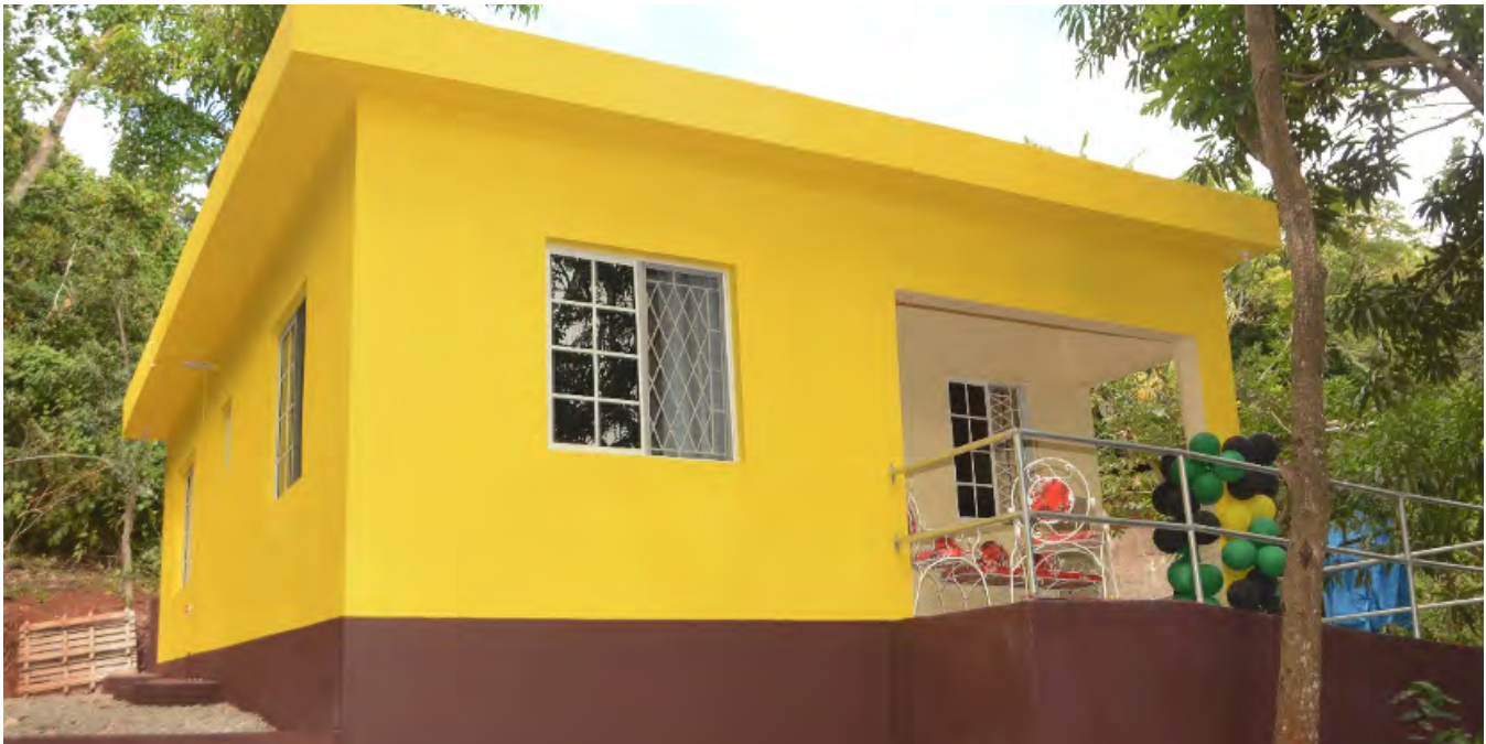
Indigent Housing Unit in Moreland Hill, Westmoreland.
