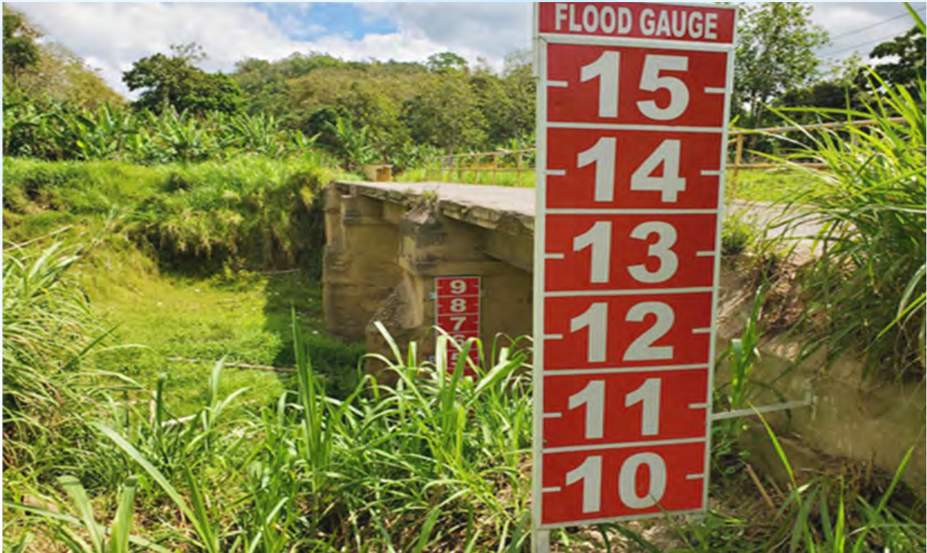
Flood gauge installed at Thatchwalk Bridge (Aenon Town).
