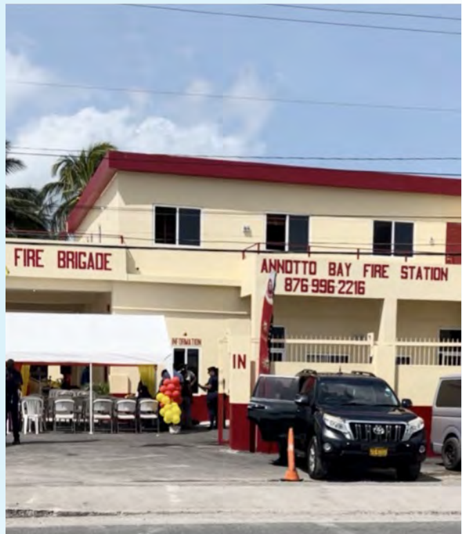
Annotto Bay Fire Station after renovation
