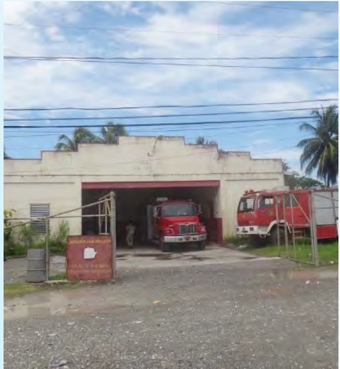
Annotto Bay Fire Station before renovation
